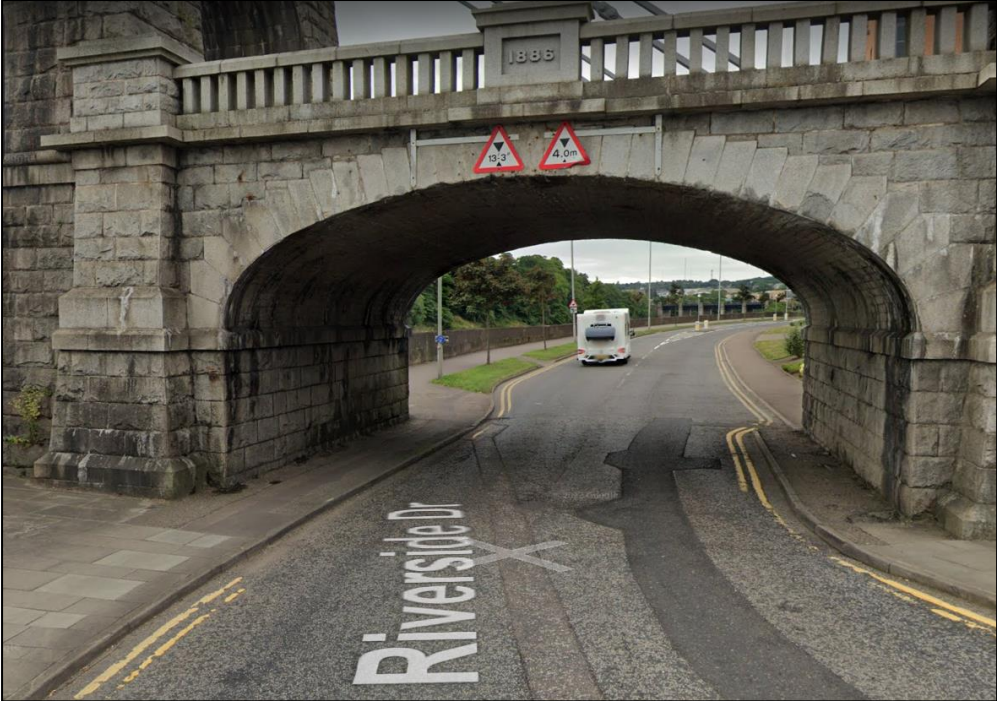
Figure 43. Road & Footway narrowing Under Wellington Suspension Bridge
