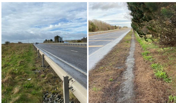
Figure 3.1: Current lack of / narrow path provision
